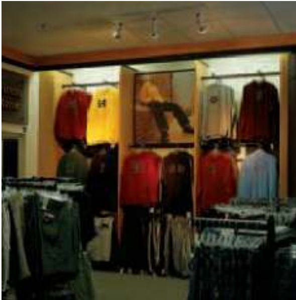
Three 90W PAR lamps using a total of 270 watts are used in this display. Spot or flood lamps need to be stocked for optimum illumination under varying conditions.
